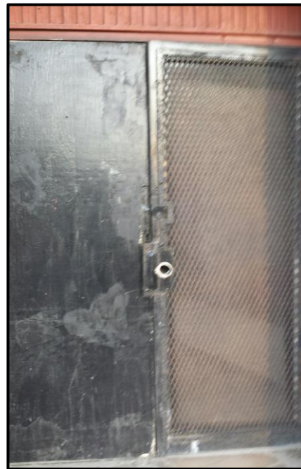
Figures 6.4 & 6.5 Missing Door Locks (1 & 2). Photo Credit: Matthew Hammer
