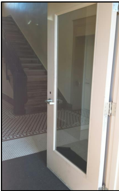
Figures 6.4 & 6.5 Missing Door Locks (1 & 2). Photo Credit: Matthew Hammer
