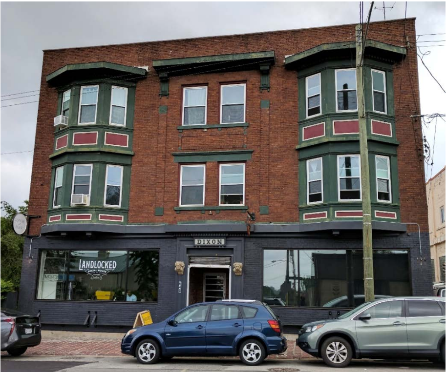
Figure 5.11. The Dixon Building circa May 2018. Photo credit: Shannon Linning
