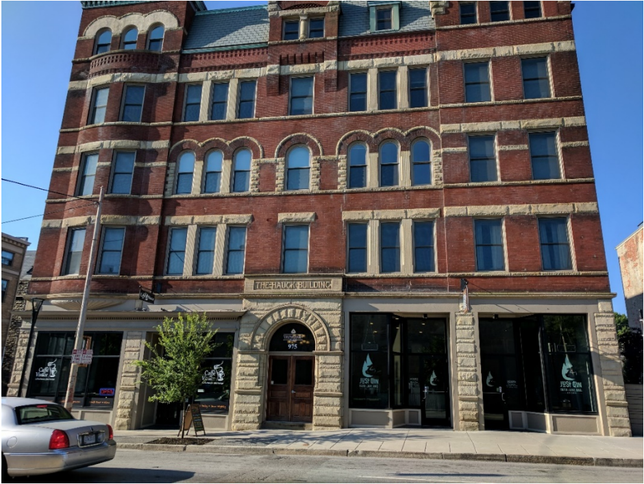
Figure 5.10. The Hauck Building circa July 2018. Photo credit: Shannon Linning
